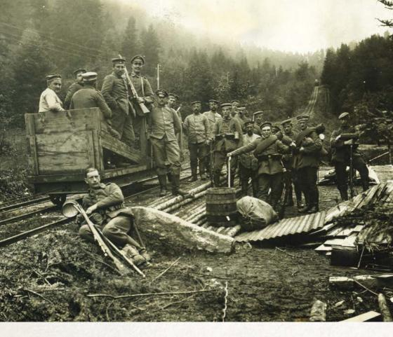
The funicular railway was one of the key elements of this military transport system. It worked with the aid of traction cables: while one trolley went up on a track, the other one went down on the second track, thereby acting as a counterweight.
