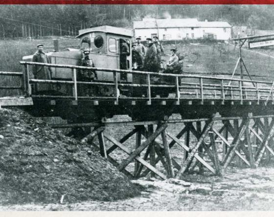
he narrow gauge railways belonged to the German transport network and were supplemented by the funicular and cable cars to transport men and equipment to the front. They could either be composed of tracks without sleepers, or consisted of rails laid on wooden or metal sleepers.
